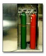
These cabinets have been designed to house gas cylinders to prevent unauthorized access to the cylinders and for the safe handling of cylinders.
